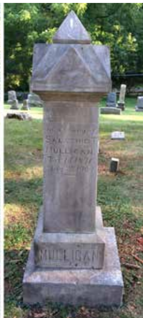
After washing with water and applying D2 - August 2016
