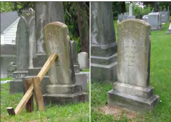
Leaning markers were supported with boards before being re-set by Lough Memorials.
